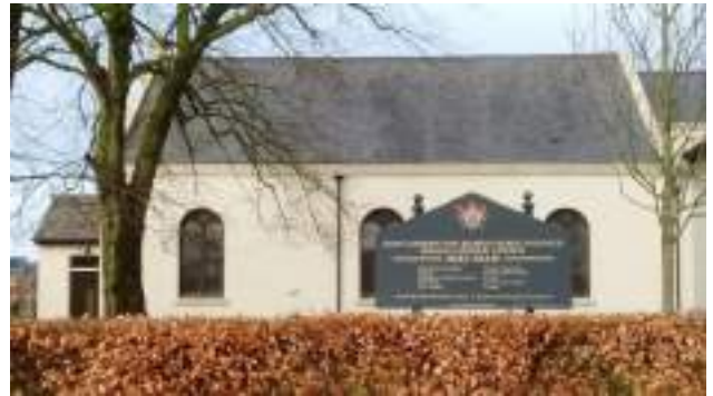
St Andrews and Blessed George Haydock Church
